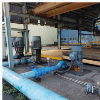
SCALE PIT泵浦功率修改
